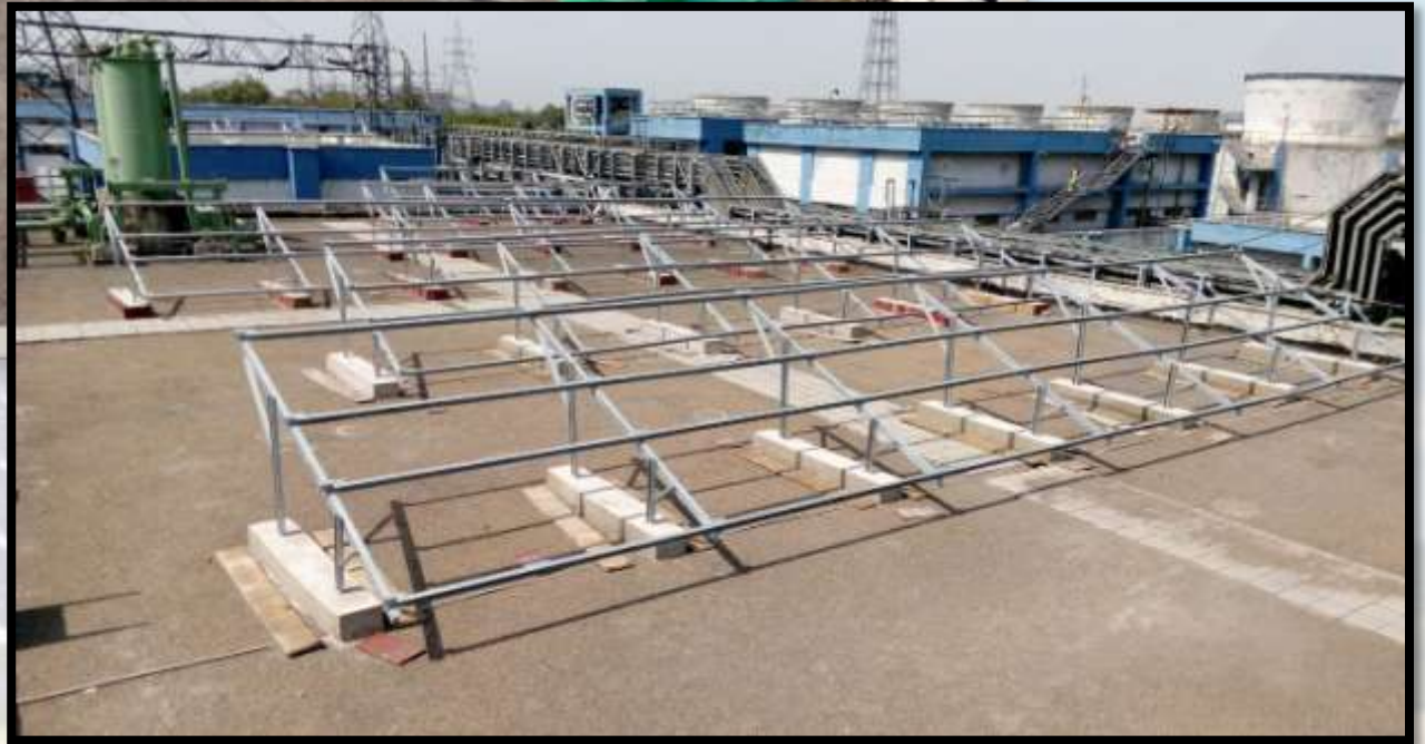
380 KW at IPGCL Gas Power Plant (Govt. Project)
