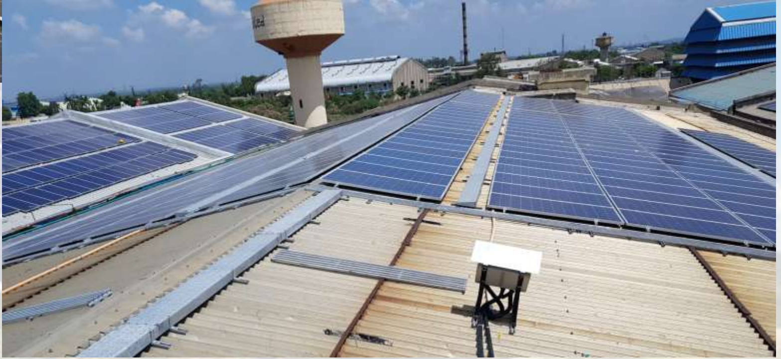
1.5 MW at LNJ Bhilwara Group, Rajasthan
